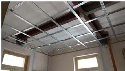
The framework for the false ceiling with the structural support (I-beams) above.
